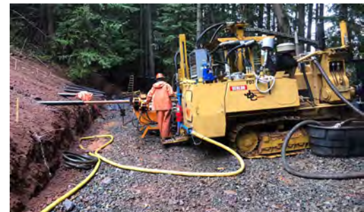
Example of a constructed horizontal drain mitigation.
