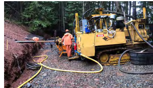
Example of a constructed horizontal drain mitigation.
