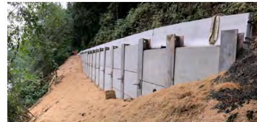
Example of a constructed soldier pile tieback wall mitigation.
