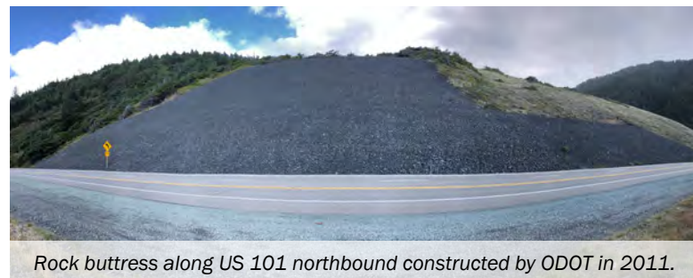
Example of a constructed shear key mitigation.
