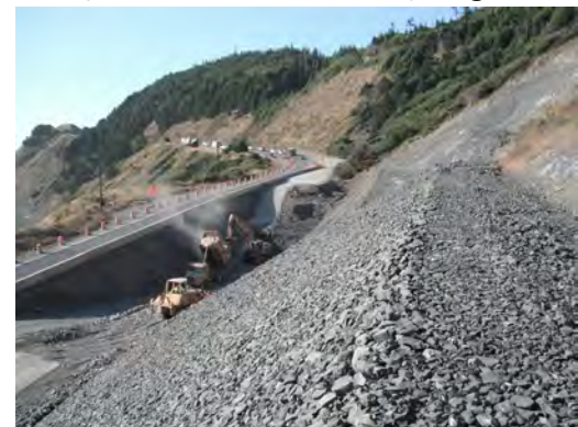
Example of a constructed shear key mitigation.
