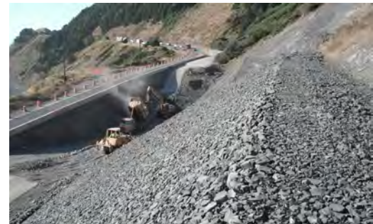
Example of a constructed shear key mitigation.
