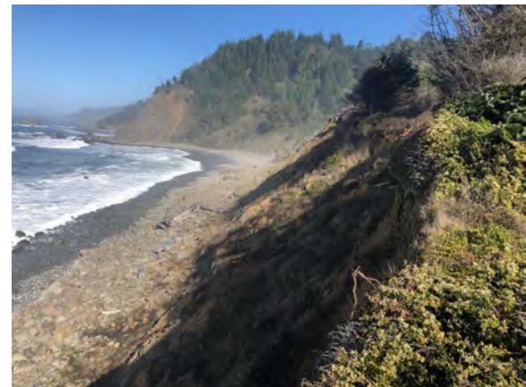
Portion of the landslide toe near the coastline that is being eroded (facing north).
